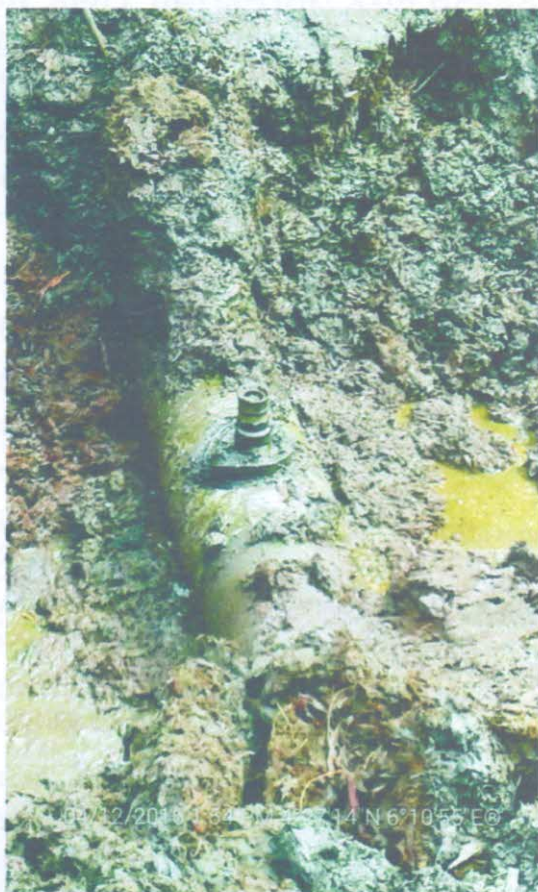
Incident Point after Excavation
