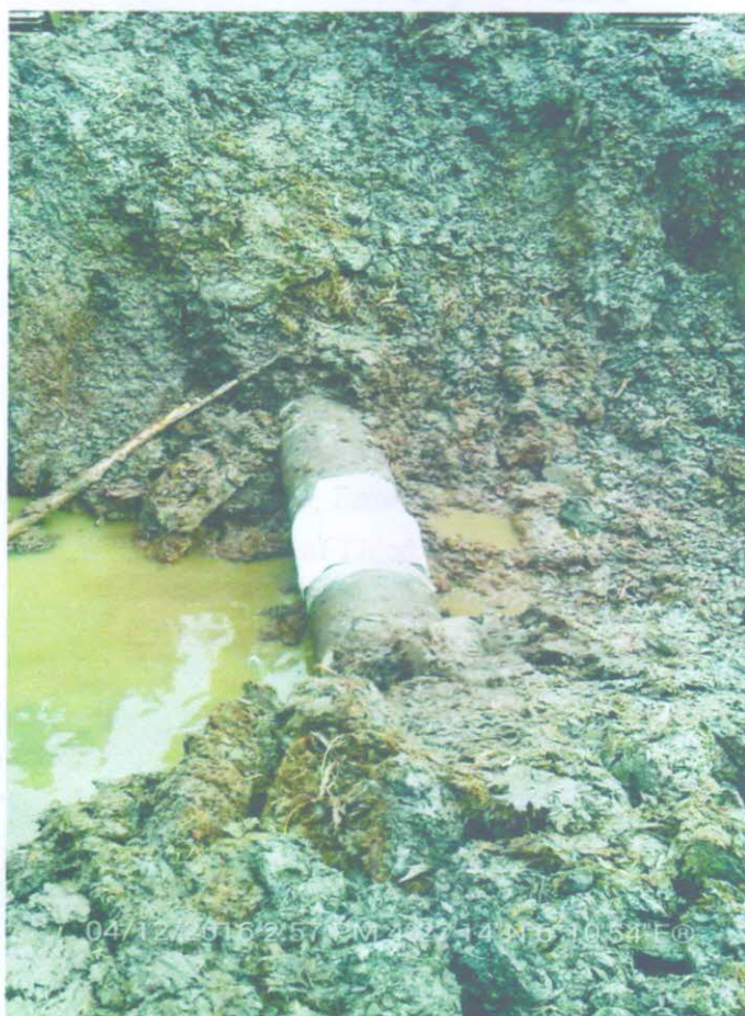
Incident Point after Repairs
